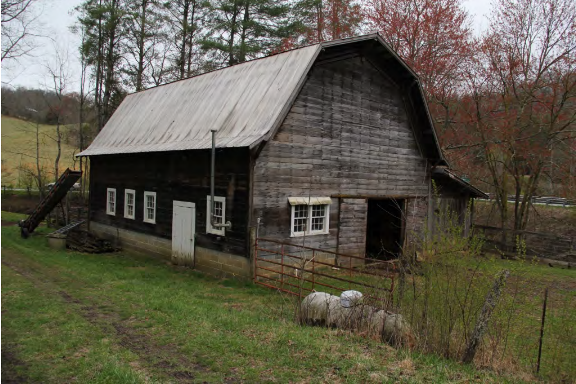
Sheep barn, oblique view to northwest
