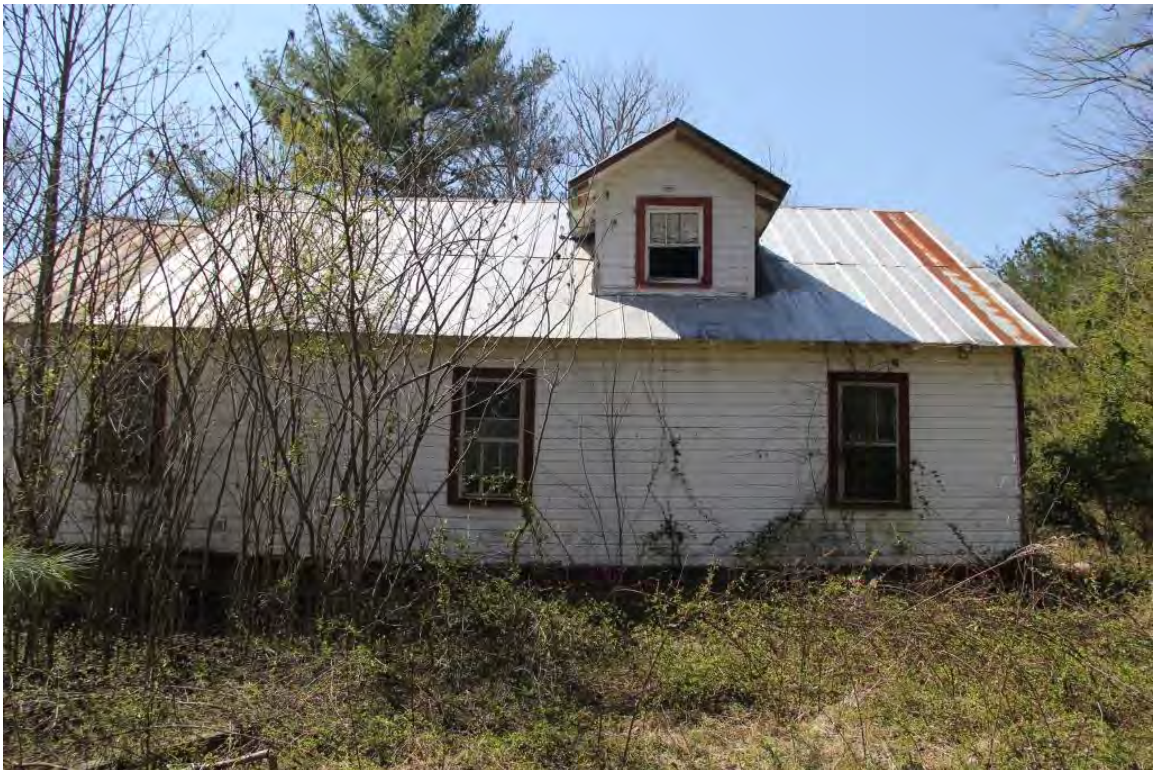
Coffey House, east elevation, view to west
