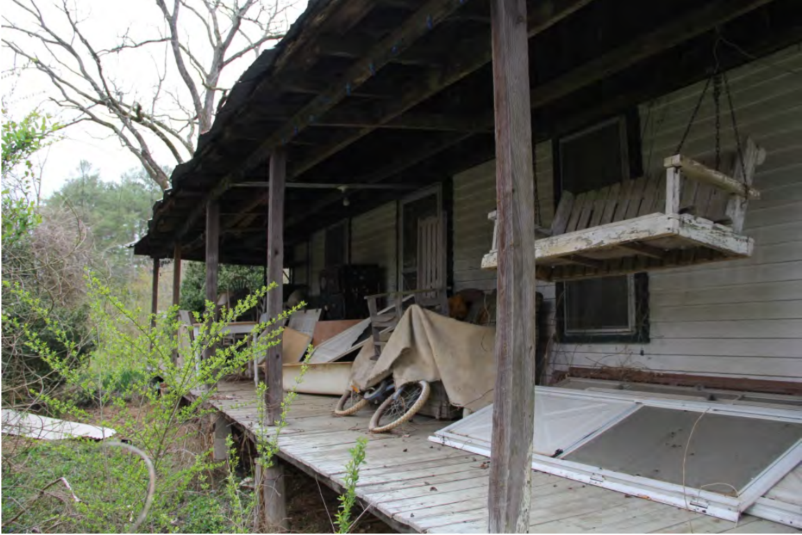
Cook-Dills House, front porch, oblique view to west
