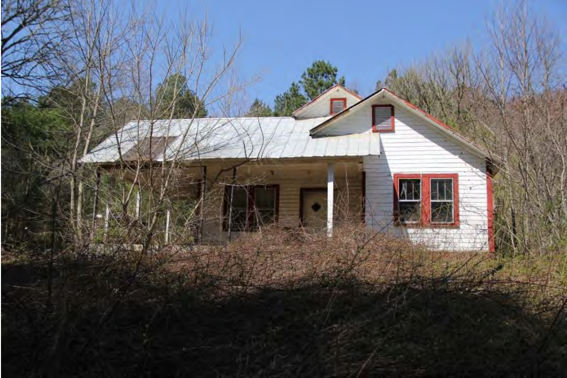
Coffey House, façade, view to north
