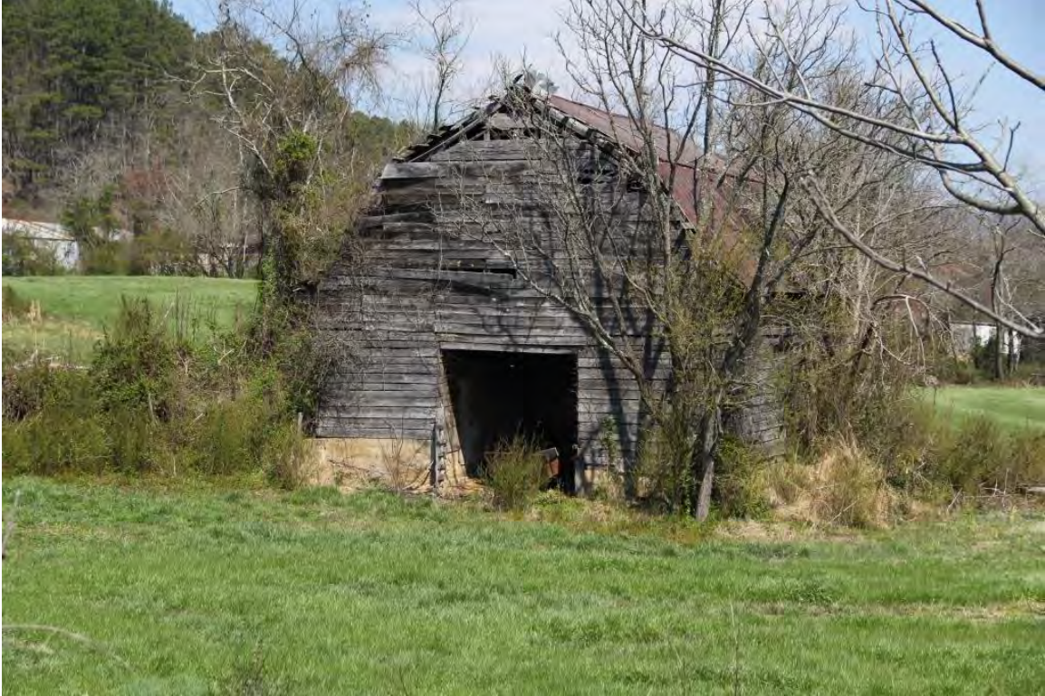
Barn, façade, view to northeast
