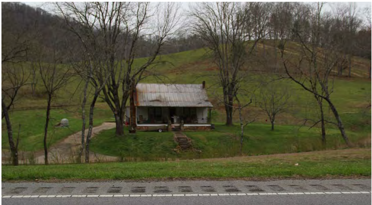
Vance and Dolly Lovin House, 4011 Hwy 64 West, main house, view to west
