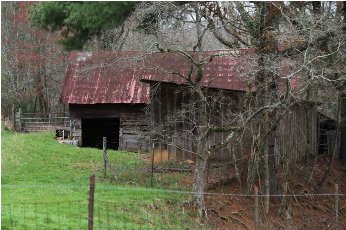
Storage shed (foreground) and barn, view to southwest
