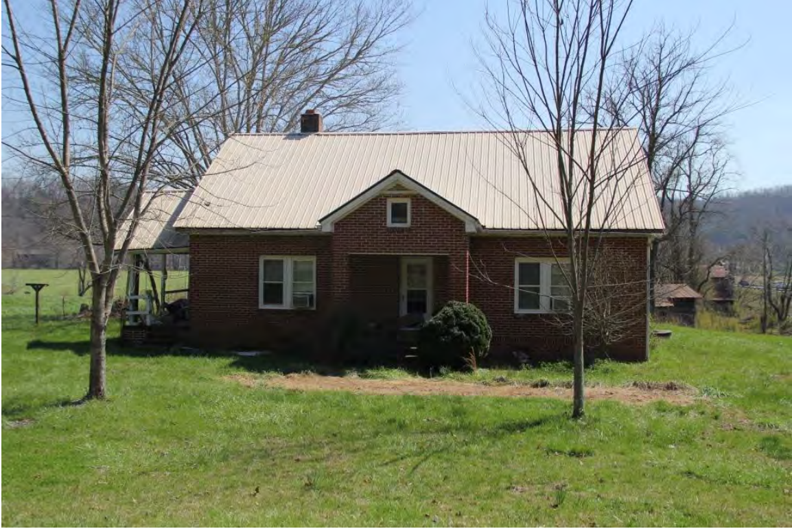
Crisp House, façade, view to southeast
