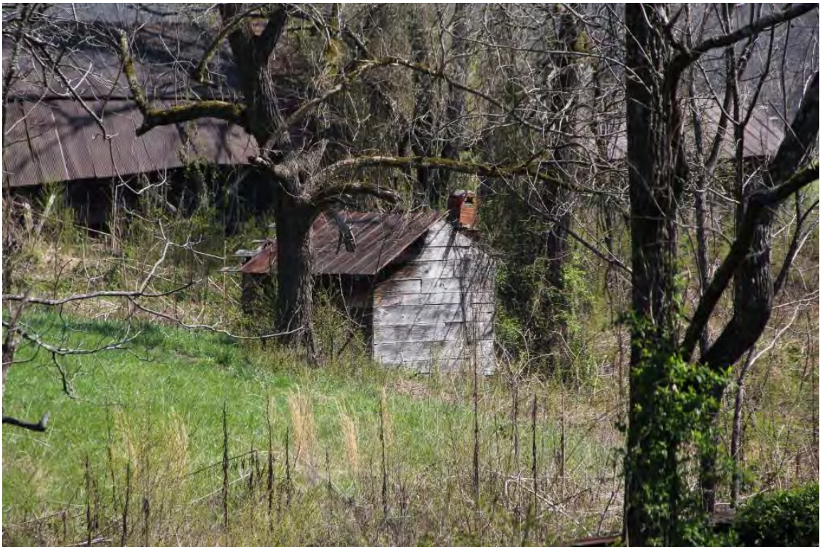
Smokehouse, oblique rear view to southeast
