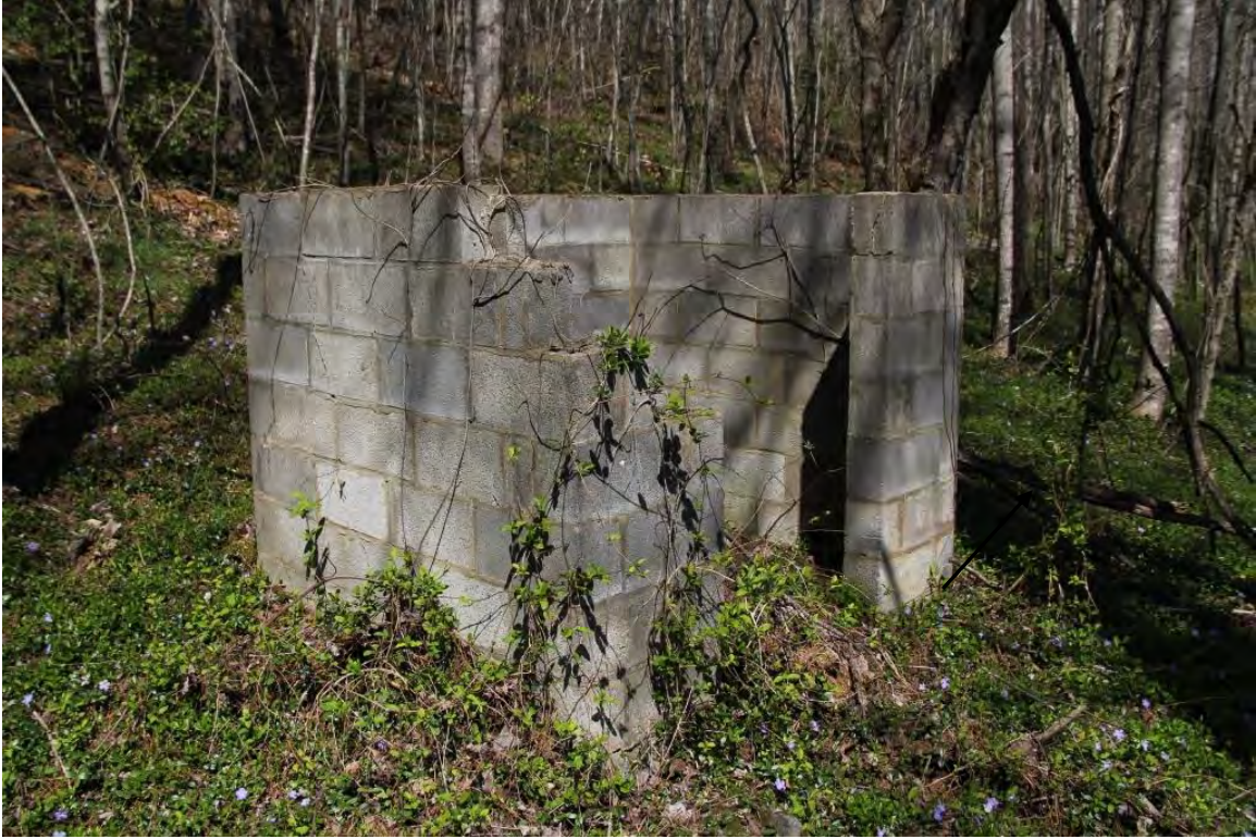
Storage building, oblique view to northeast
