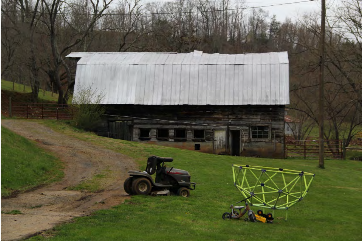
Barn, south elevation, view to north
