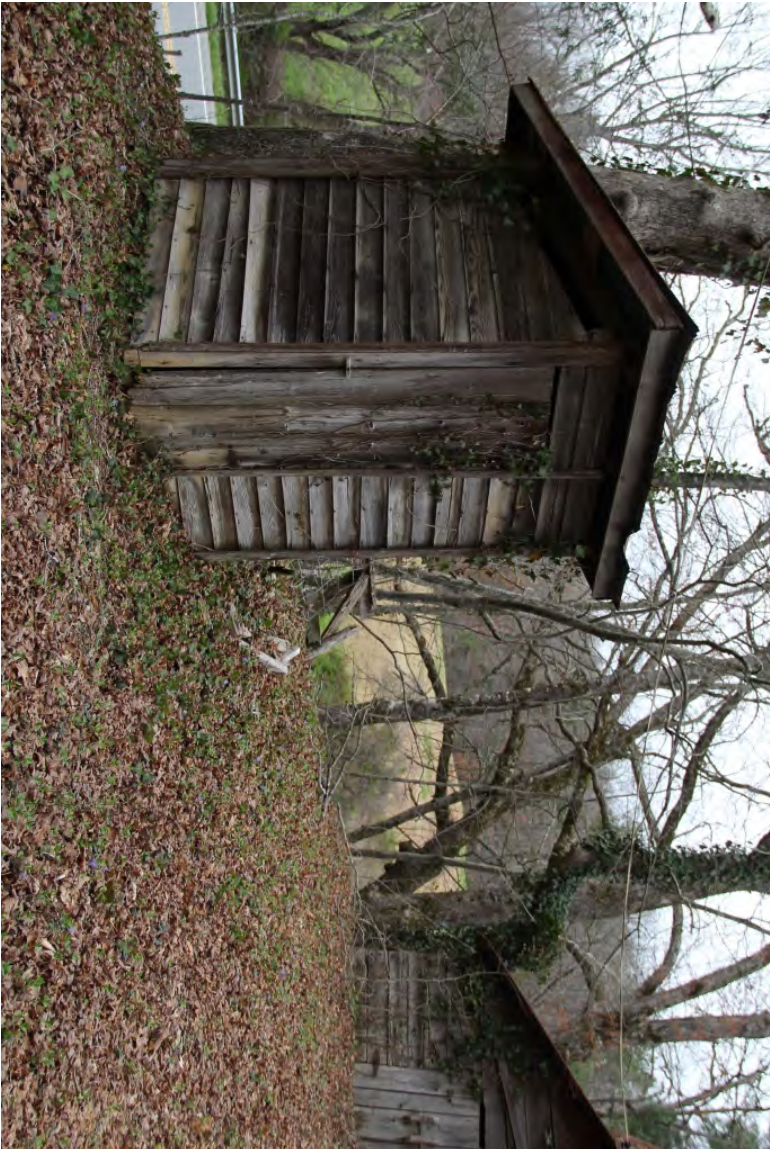
Privy, view to northeast
