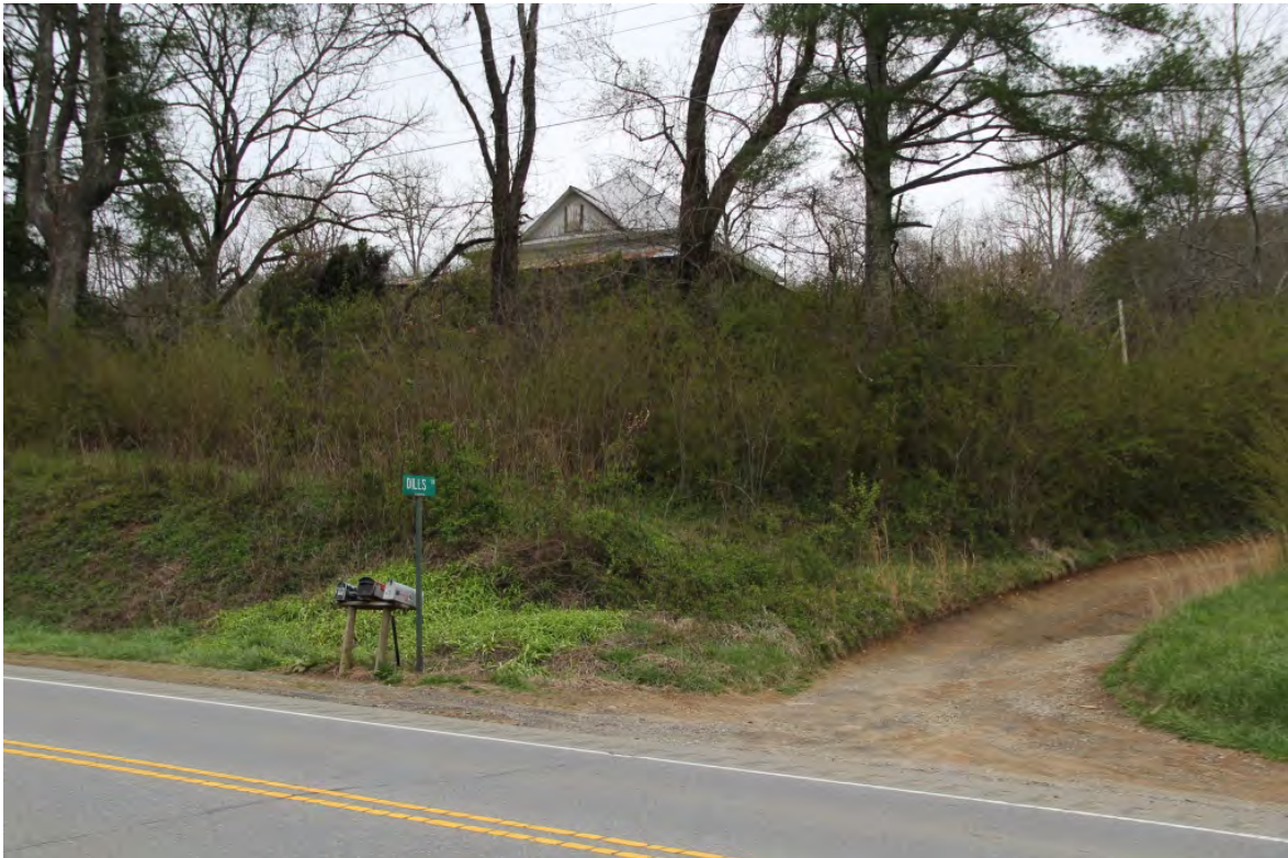
Cook-Dills House, 96 Dills Lane, overall view to northwest from US 64W
