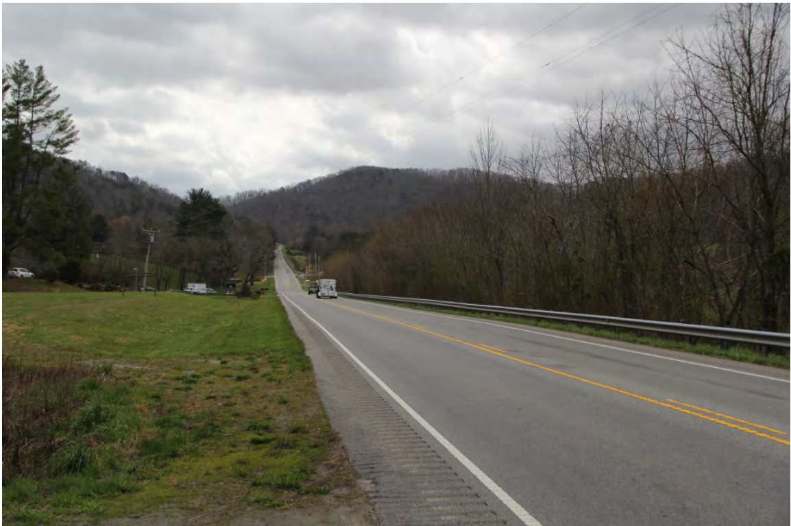
US 64 W, view southeast to Sweetwater Gap
