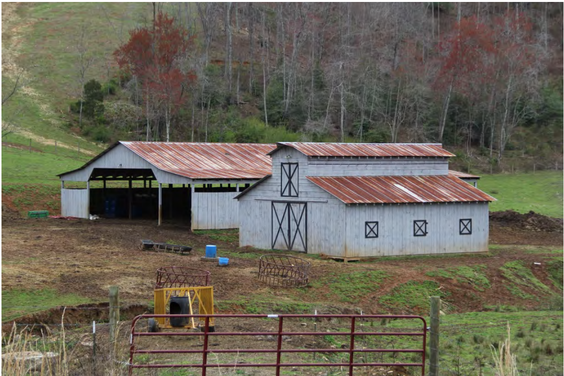
Barns (ca. 2014), oblique view to northwest
