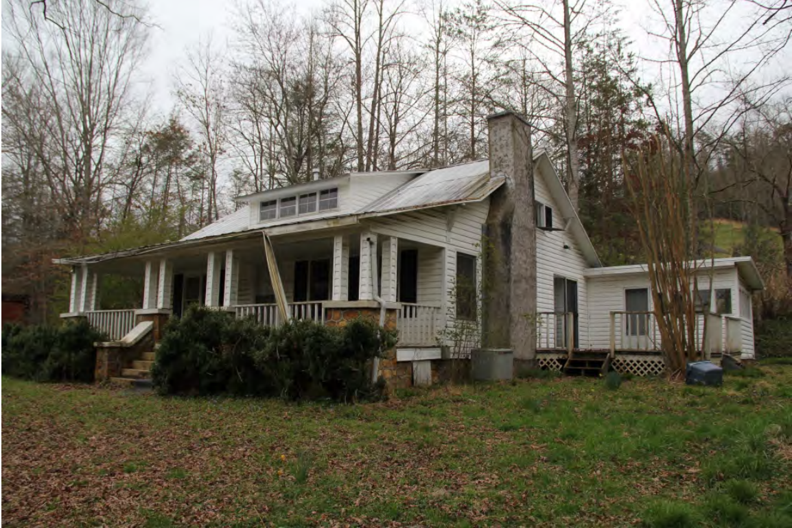
Anderson House, oblique front view to west
