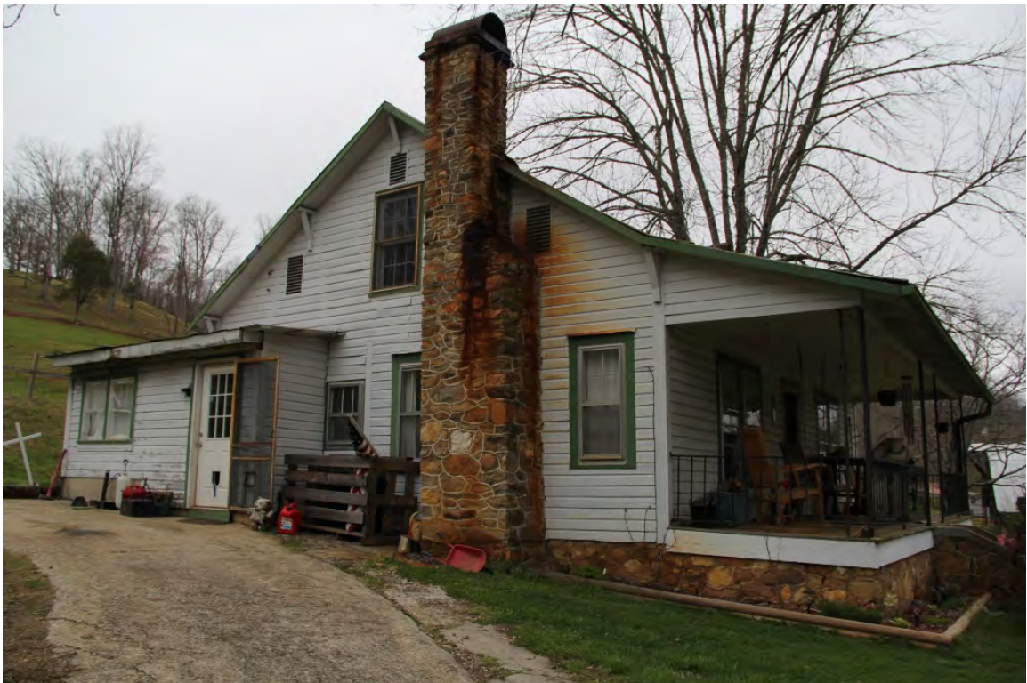
Lovin House, south elevation, view to north
