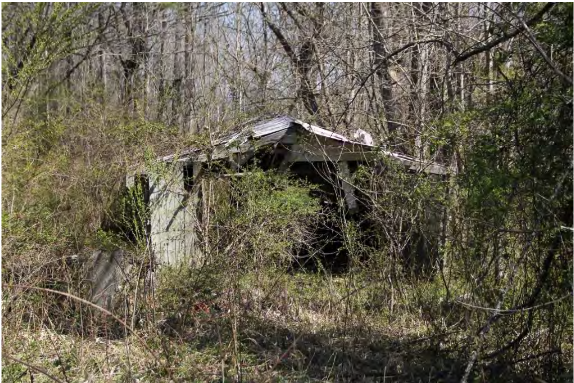
Garage, façade, view to east
