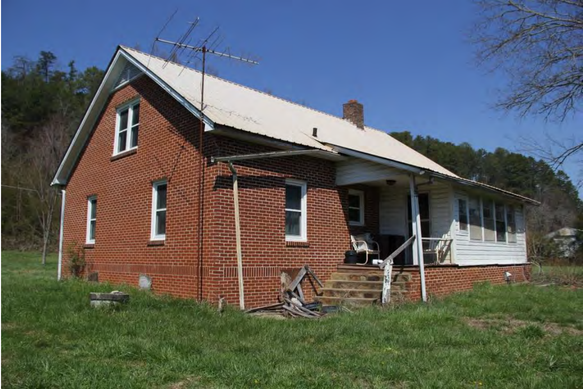
Crisp House, oblique rear view to northwest
