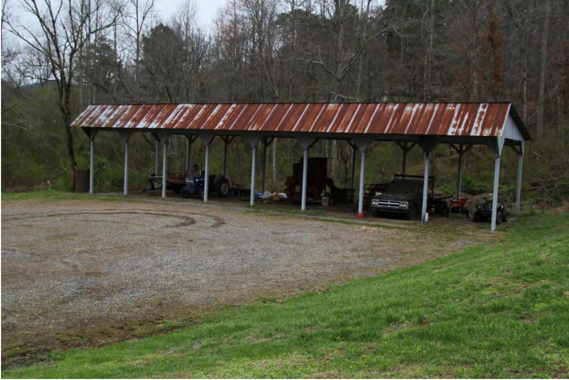
Vehicle shed (ca. 2014), view to south
