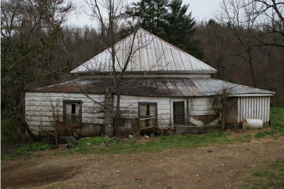
Cook-Dills House, rear elevation, view to south
