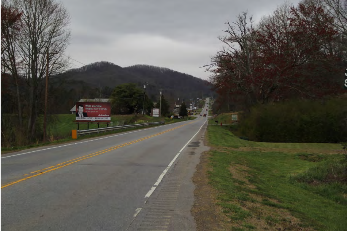
Project beginning, view to southwest along US 64 W, west of Hayesville
