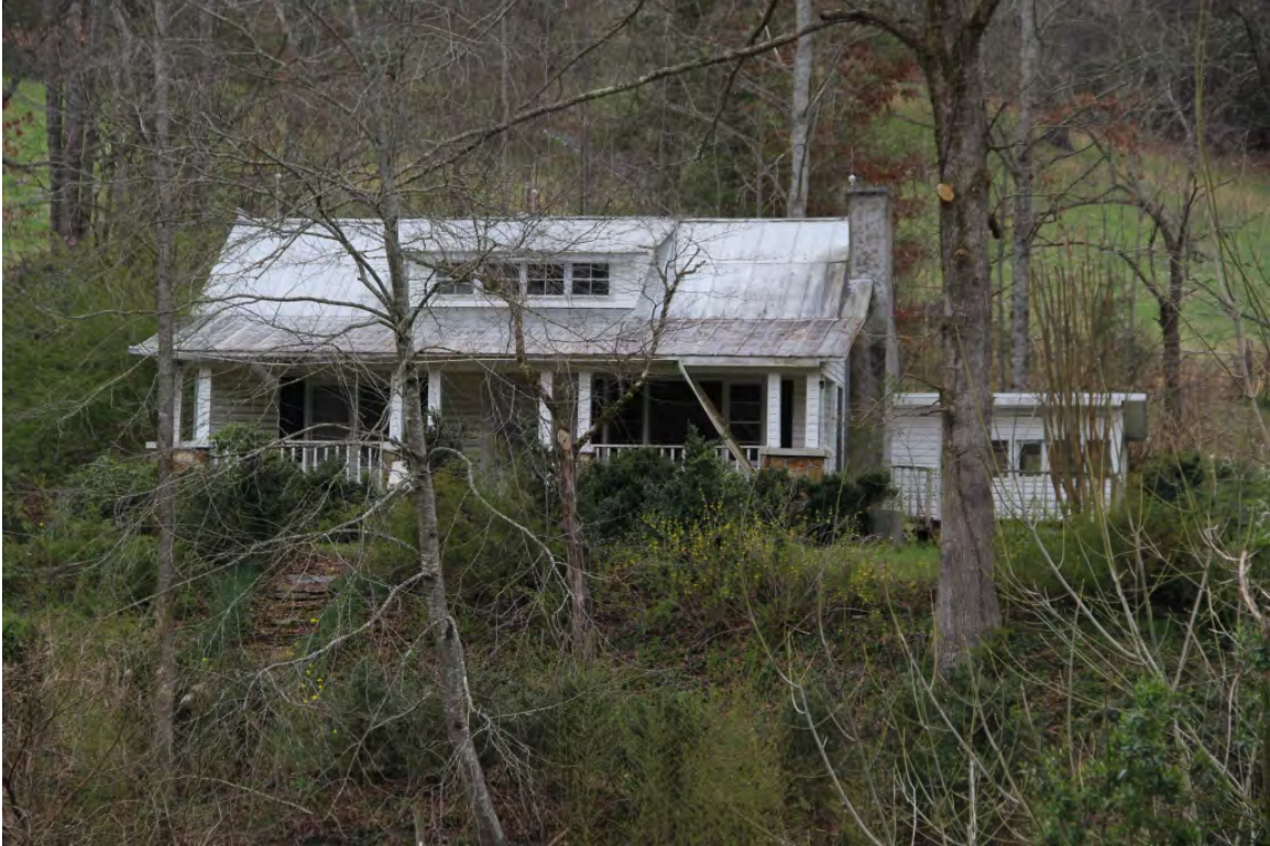
Anderson House, view to southwest
