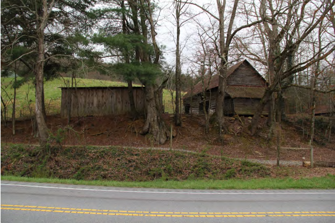
Storage shed (l) and barn (r), view to south
