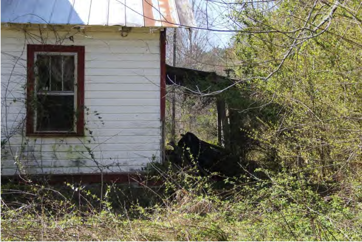
Coffey House, rear porch, view to west
