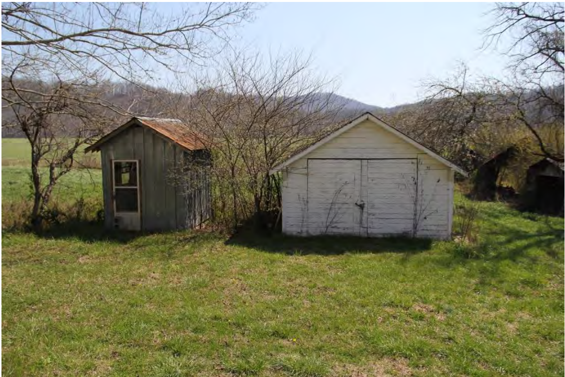
Garden shed (l) and garage (r), view to southeast
