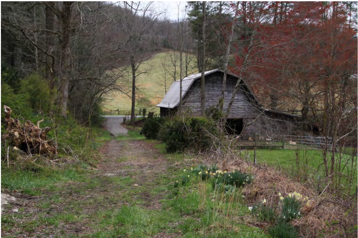
Sheep barn and old highway roadbed, overall view to southwest
