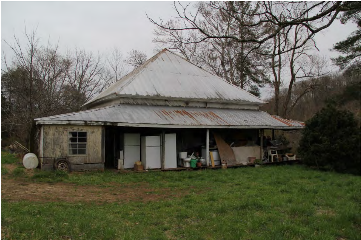
Cook-Dills House, west elevation, view to east
