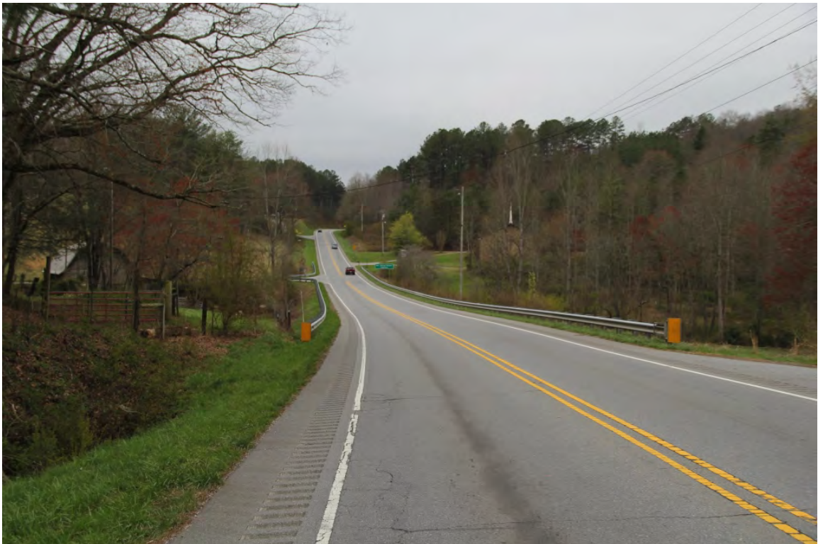
US 64 W, view southwest to intersection with Stewart Cove Road (SR 1130)
